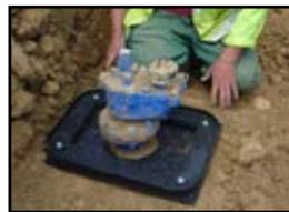
The chamber can be easily installed over existing valves using the split base.
